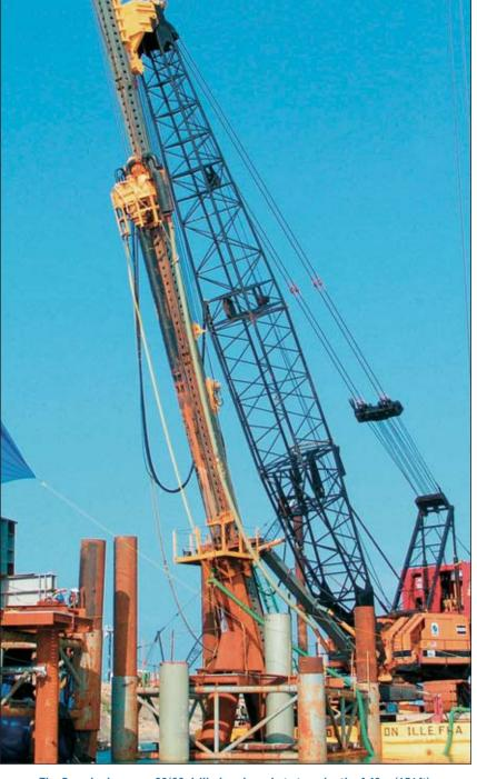
The Berminghammer 60/60 drilled rock sockets to a depth of 46m (151ft).
