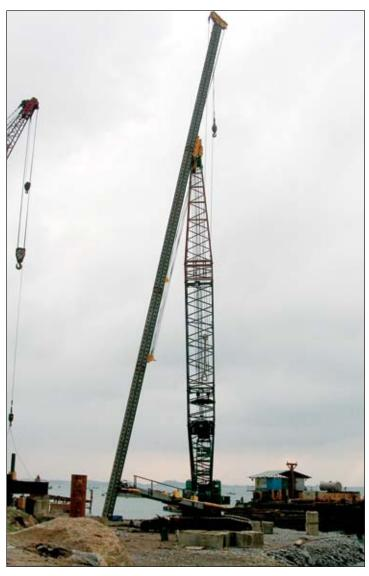
The L23 lead system, drilling six piles a day on a project in Vietnam. One of the obstacles to overcome was the distance from the crane that drilling had to take place. Bermingham designed and fabricated a 7.6m (25ft). three-stage spotter so the client could work at more than a 15m (50ft) radius from the center of the crane.
